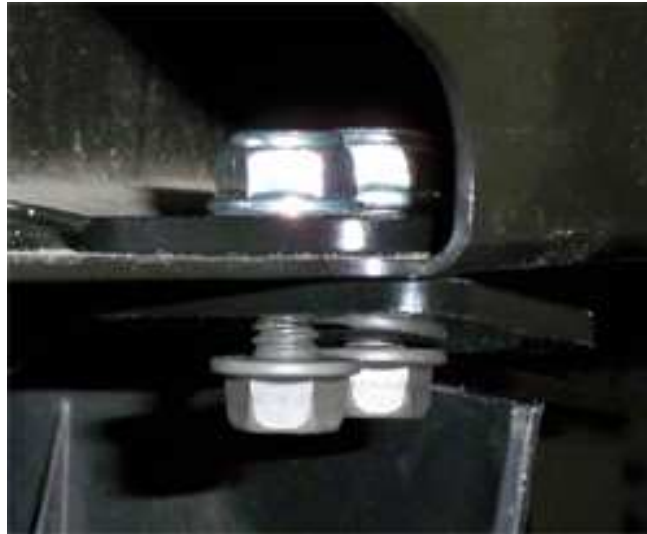
\frac{3}{4} " bolt, bracket, bumper support, slotted tab, capped off with locknut
